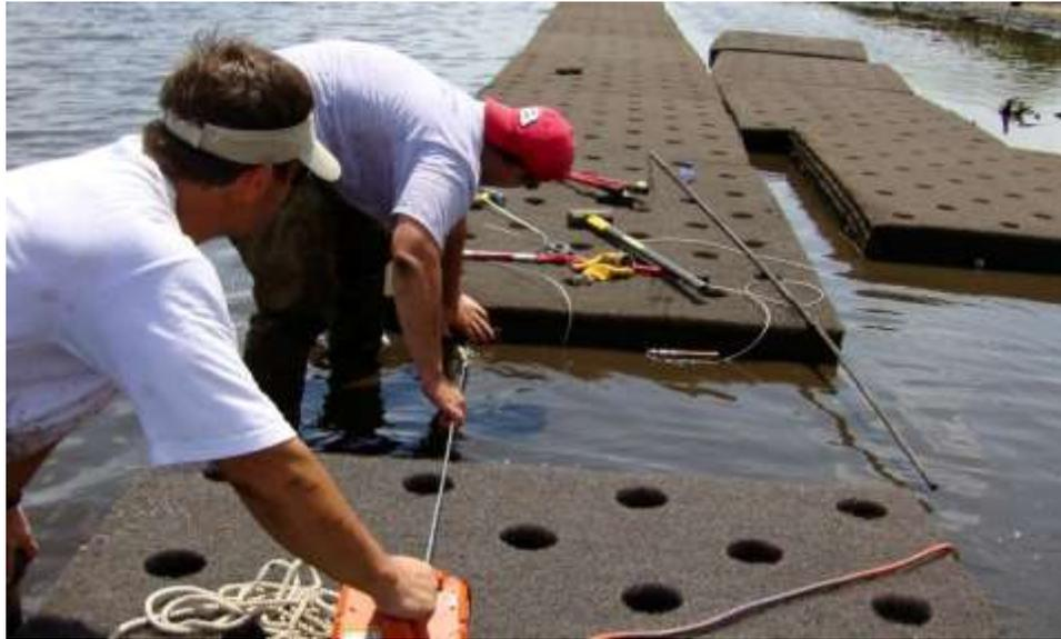
*BioHavens being installed at Bayou Sauvage National Wildlife Refuge near New Orleans to protect an eroding shoreline by allowing sediments to accumulate and by providing new vegetation. August 2009*
