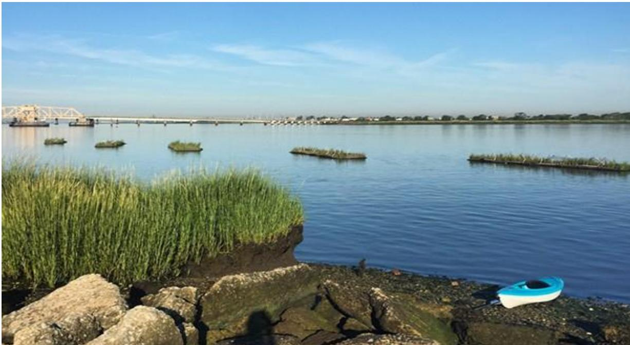
Five attenuators, each approximately 40 feet in length were anchored to the seabed approximately 100 feet off-shore. The attenuators were angled to deflect waves produced from prevailing northeast winds
