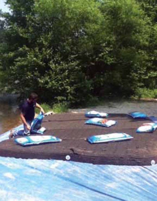
Figure 1. Construction of the floating wetland islands at Westtown Lake.
