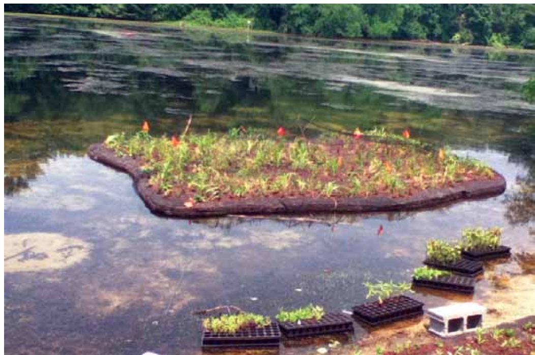
Figure 3. Positioning one of the floating wetland islands on Westtown Lake.
